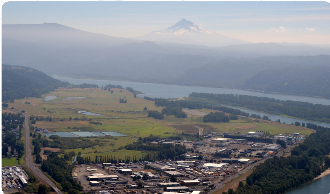
This photo is looking east. In the forefront is the Port of Camas-Washougal's Industrial Park and the City of Washougal's wastewater treatment plant. In the back is the Refuge and the Columbia River.
